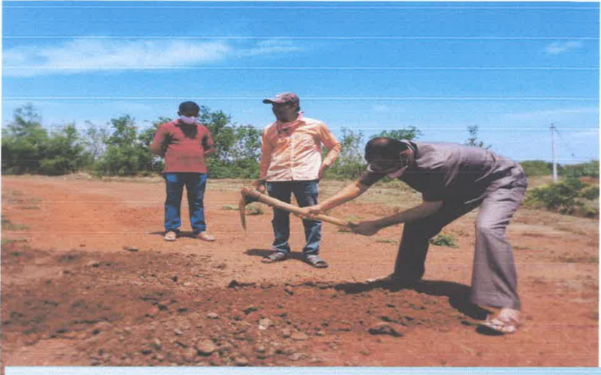
Disposal Pit for Bio-medical Waste
